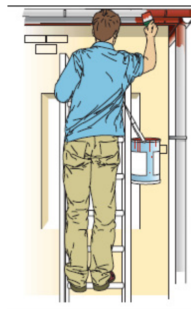
Maintaining 3 points of contact
